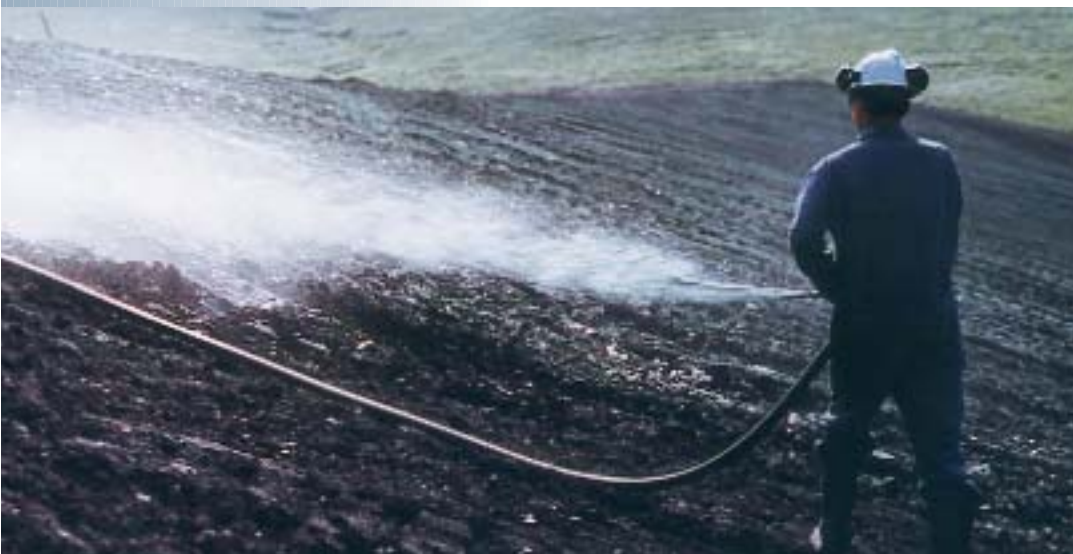
Hydroseeding a mine waste slope. The spray contains grass seed, fertilizer and a natural agent to help the seed stick to the ground. Hydroseeding is an important part of ongoing reclamation activities at the mine.
