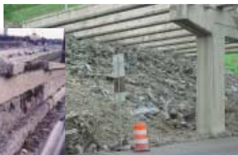
Effect of corroding reinforcing steel
